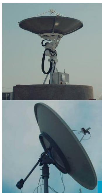
Επάνω: X-/L- band acquisition station, Κάτω: MSG SEVIRI acquisition station.
